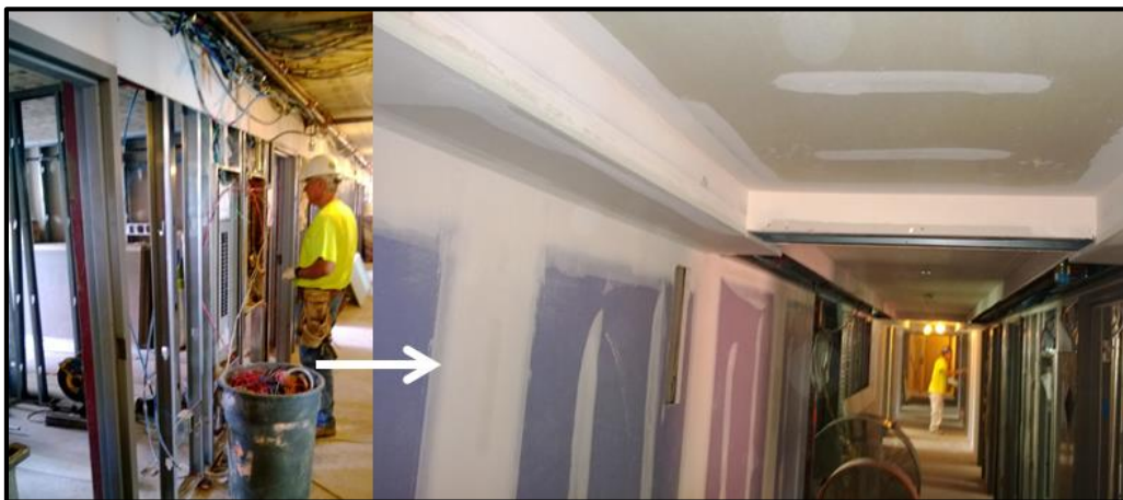
Figure 7: MEP coordination and bulkhead in typical corridor | Quaid Spearing
